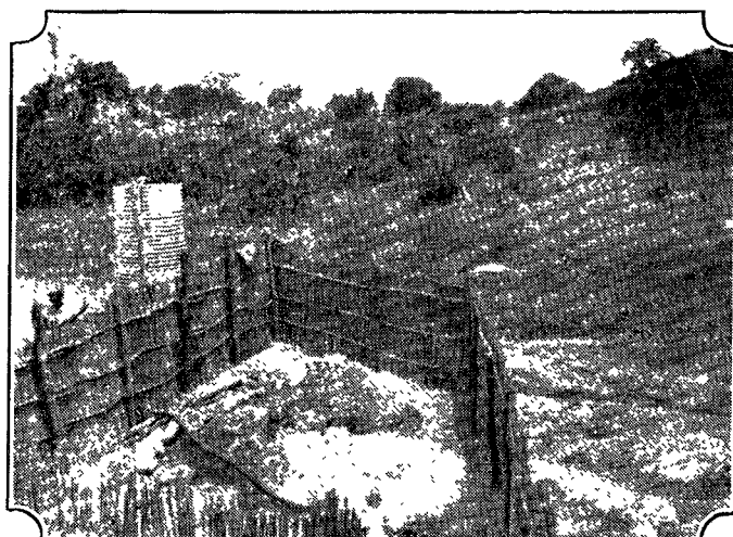
FIG. 2.—Well-protected "spring" water-supply at Summit, East Africa, showing hose leading to water-tank.
